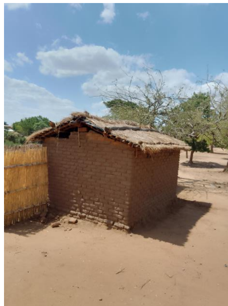
Picture 3 A house in Chapananga village reinforced with logs and rope
